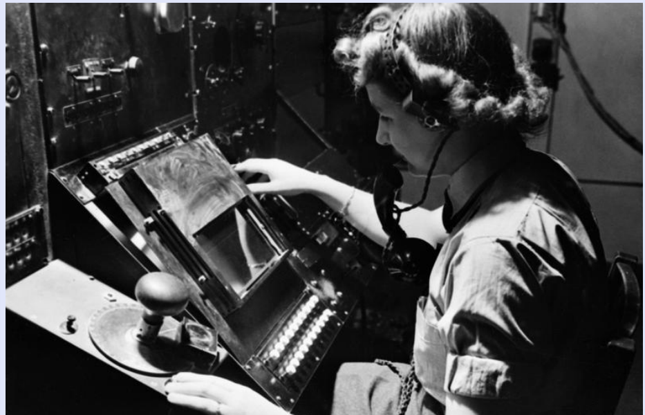
▶ A British volunteer operating a Chain Home radar position in 1940. Her right hand turns a wooden dial to determine the exact azimuth of the target.
