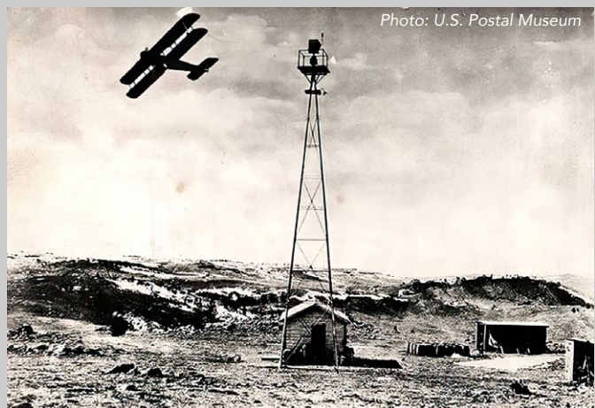
➤ Photo: One of the U.S. Army line of rotating beacons set up in Wyoming in 1921 to help pilots navigate the mail route from Dayton Ohio.
